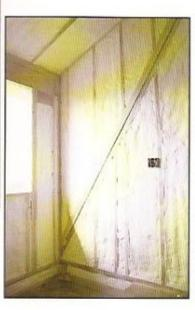
After the insulation is sprayed in place, the foam must be protected by an approved 15 minute thermal barrier.
